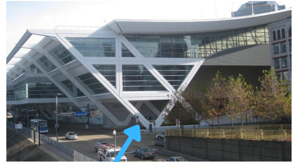
Loading Dock Entrance
